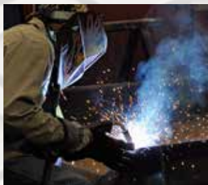
WELDING – Robotic, semi-automatic and manual including TIG and MIG
